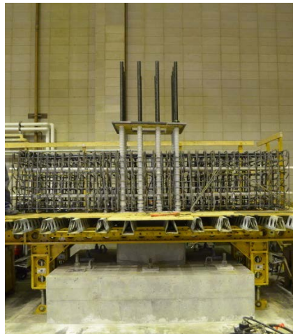
Figure 3.15: Cap beam set in place on platform over column bars
