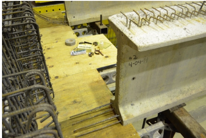
Figure 3.18: ESSP connection prior to cutting one strand and attaching anchor plates and chucks
