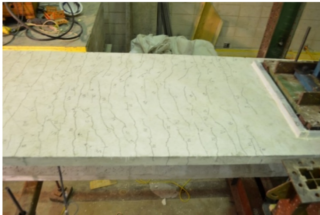
Figure 4.7: Extended deck cracking
