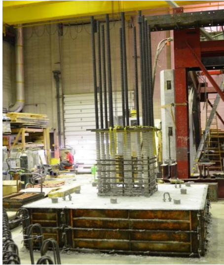
Figure 3.13: Footing and Column pour
