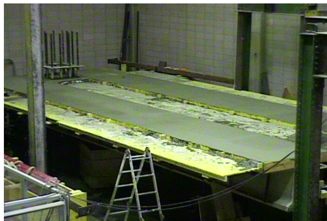
Figure 3.21: Completed cap and deck concrete pour
