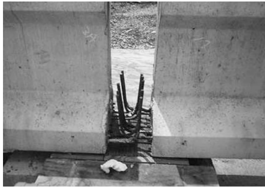
Figure 2.27: Bent reinforcing bar connection (NCHRP, 2004)
